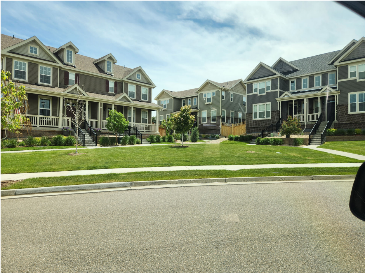
Example of trees needing replaced - in tract Y
